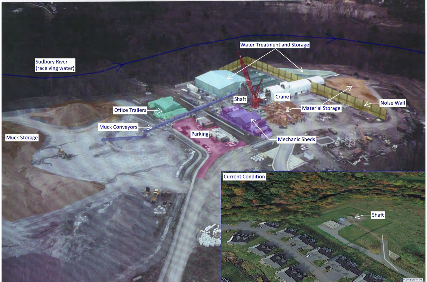
Launching Shaft site for the MWWST
