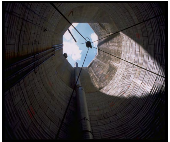
MWRA's MetroWest Water Supply Tunnel Launch Shaft from Below
